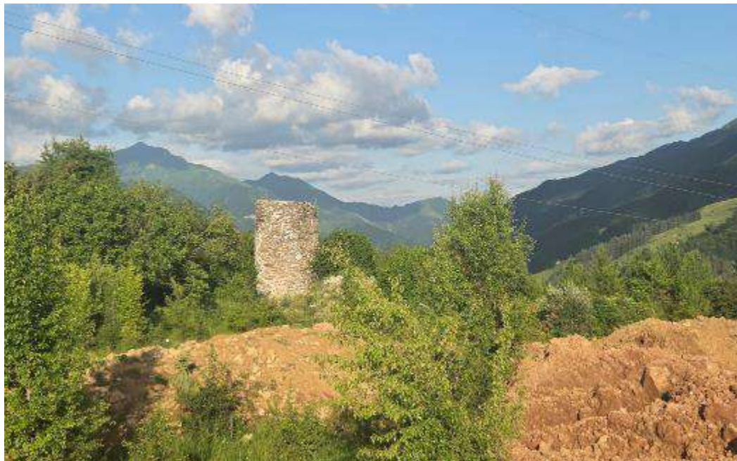
Figure 25: Gas Pipeline Relocation Works near Didveli Backed Tower (CH Site #10)
