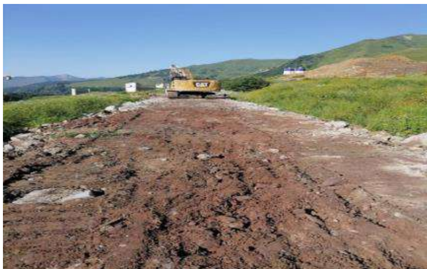
Figure 34: Improving the access road to Village Mughure
