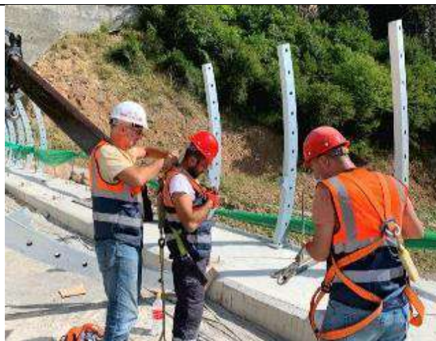
Pic 8 Inspection of fall arrest equipment at Bridge 2, LOT 2.
