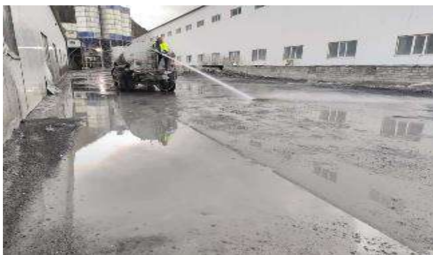
Figure 36: Washing of the Batching Plant- Kobi
