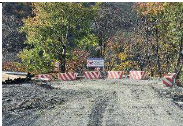
Pic 14 Edge protection at access road to Bridge 3 P19 worksite.
