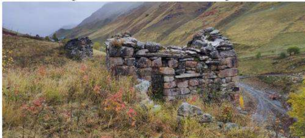
Figure 6: Measurement Point – VM#5 – Cultural Heritage #29
