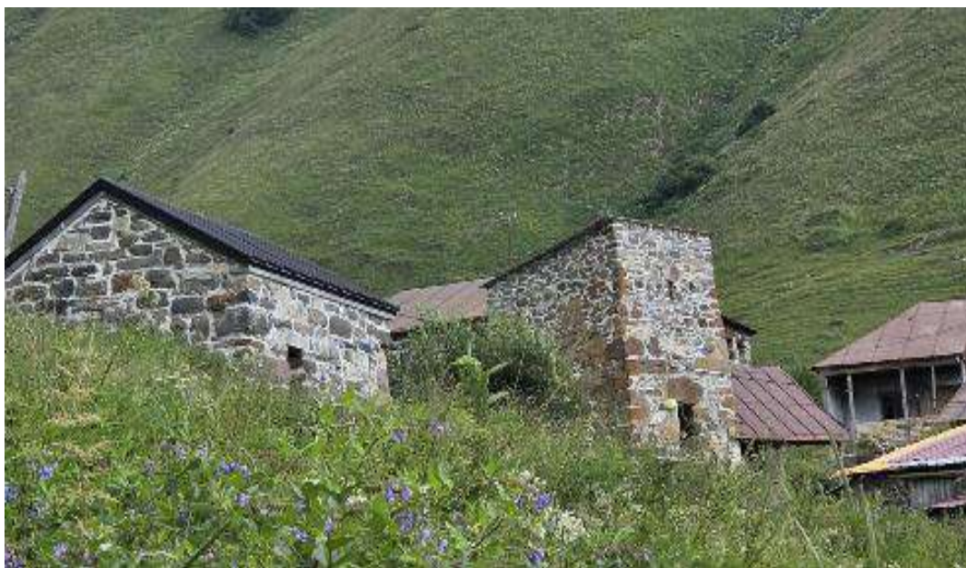
Figure 28: CH 10, conservation work completed.
