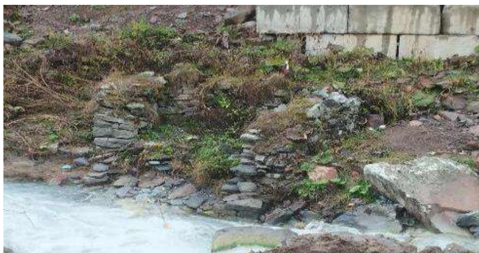
Figure 24: CH 28 being affected by the river diversion
