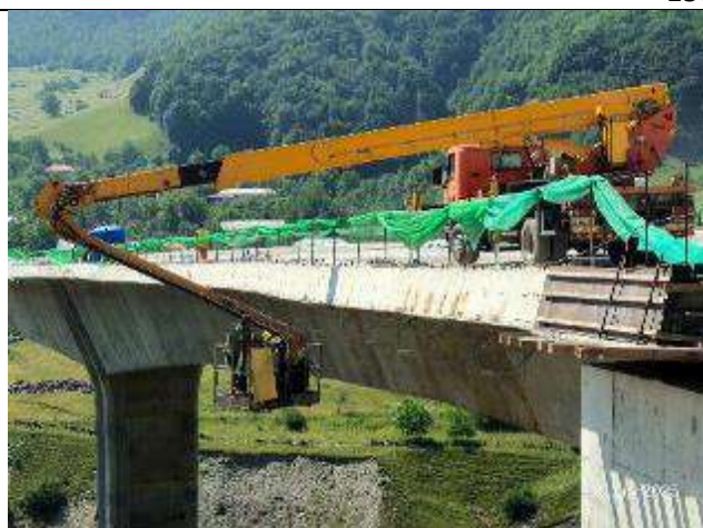
Pic 12 Improved guardrail systems at Bridge 3, A1-P3 section.
