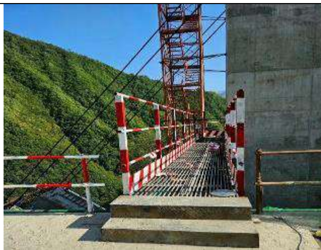
Pic 14 Edge protection at access road to Bridge 3 P19 worksite.
